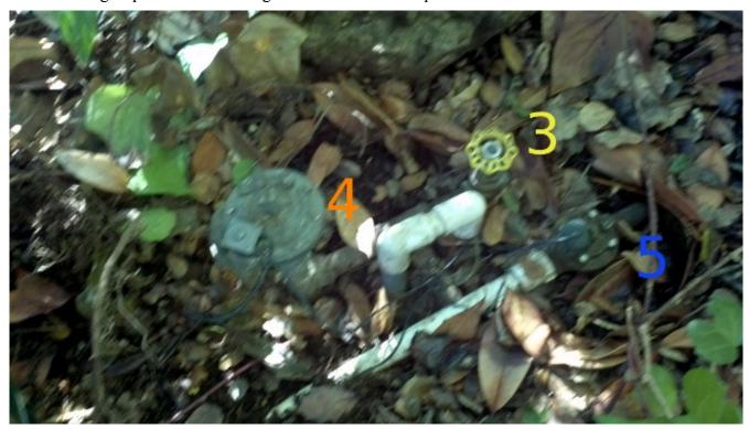
Number 4 is an electric valve (station 1) that operates two rain birds over the ivy bordered by the road, the drive way and the stone walk/stairs in front of the south end of the house. Number 5 is an electric valve (station 2) that operates 2 rain birds; one of which is just inside of the fence corner located at the south corner of the property; the other is along the fence just a short distance north west of the first.
