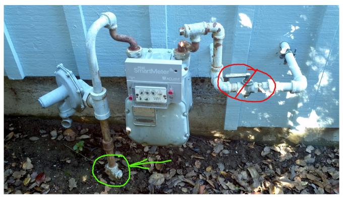
The valve near the ground circled in green is the main shut off valve. The operable part of the valve is shown below by the red arrow. A wrench is required to operate the valve.
